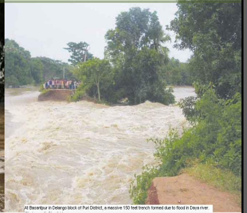
At Besatpur in Debagpur block of Puri District, a massive 150 feet breach formed due to flood in Daya river.
